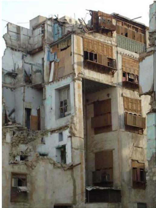
**Figure 6. View showing one example of a deteriorating residential building. It is also marked with serious cracks.**
